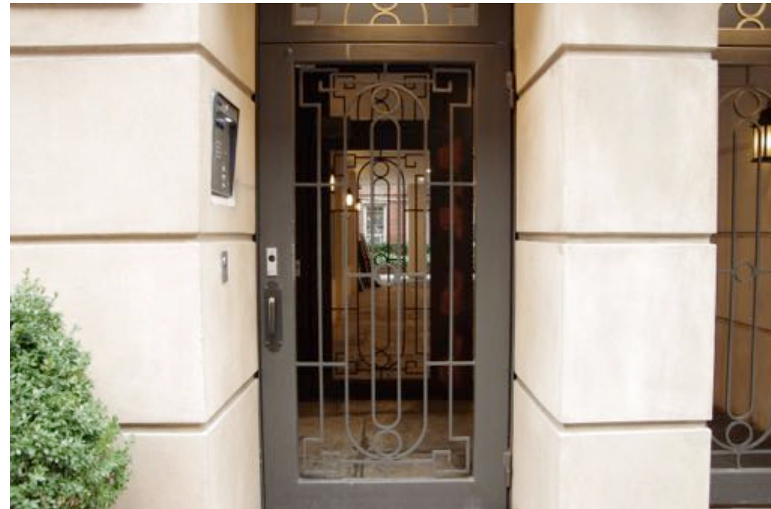
3 EXISTING VIEW OF FRONT GATE TO EXIT PASSAGEWAY
