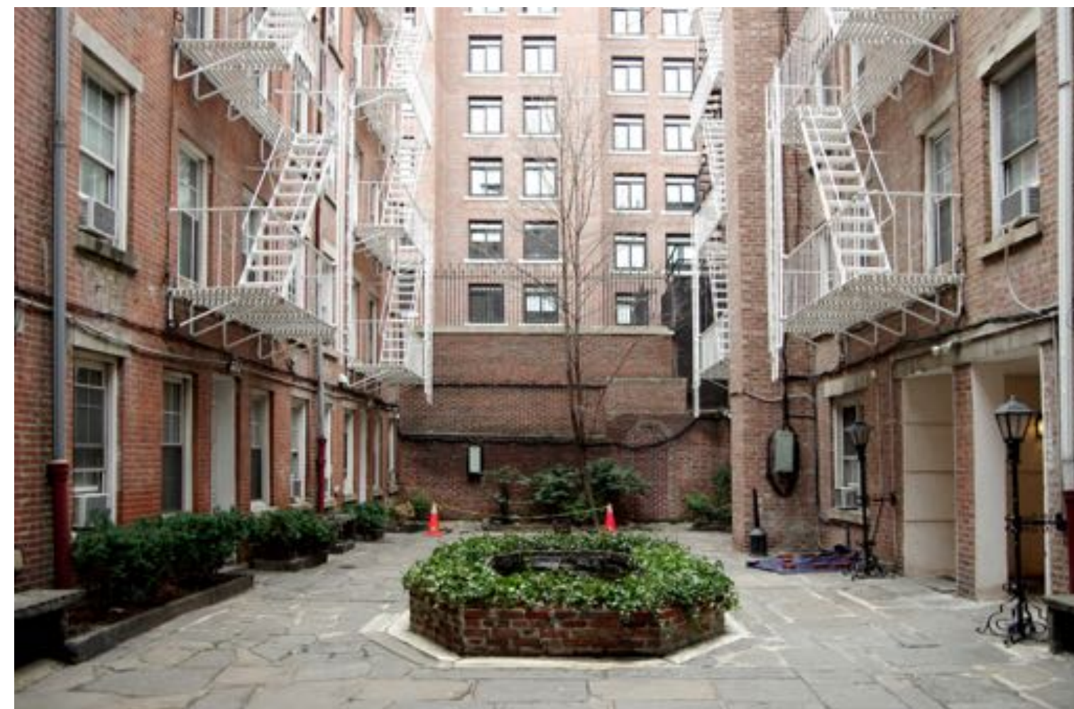
5 EXISTING VIEW OF COURTYARD LOOKING NORTH
