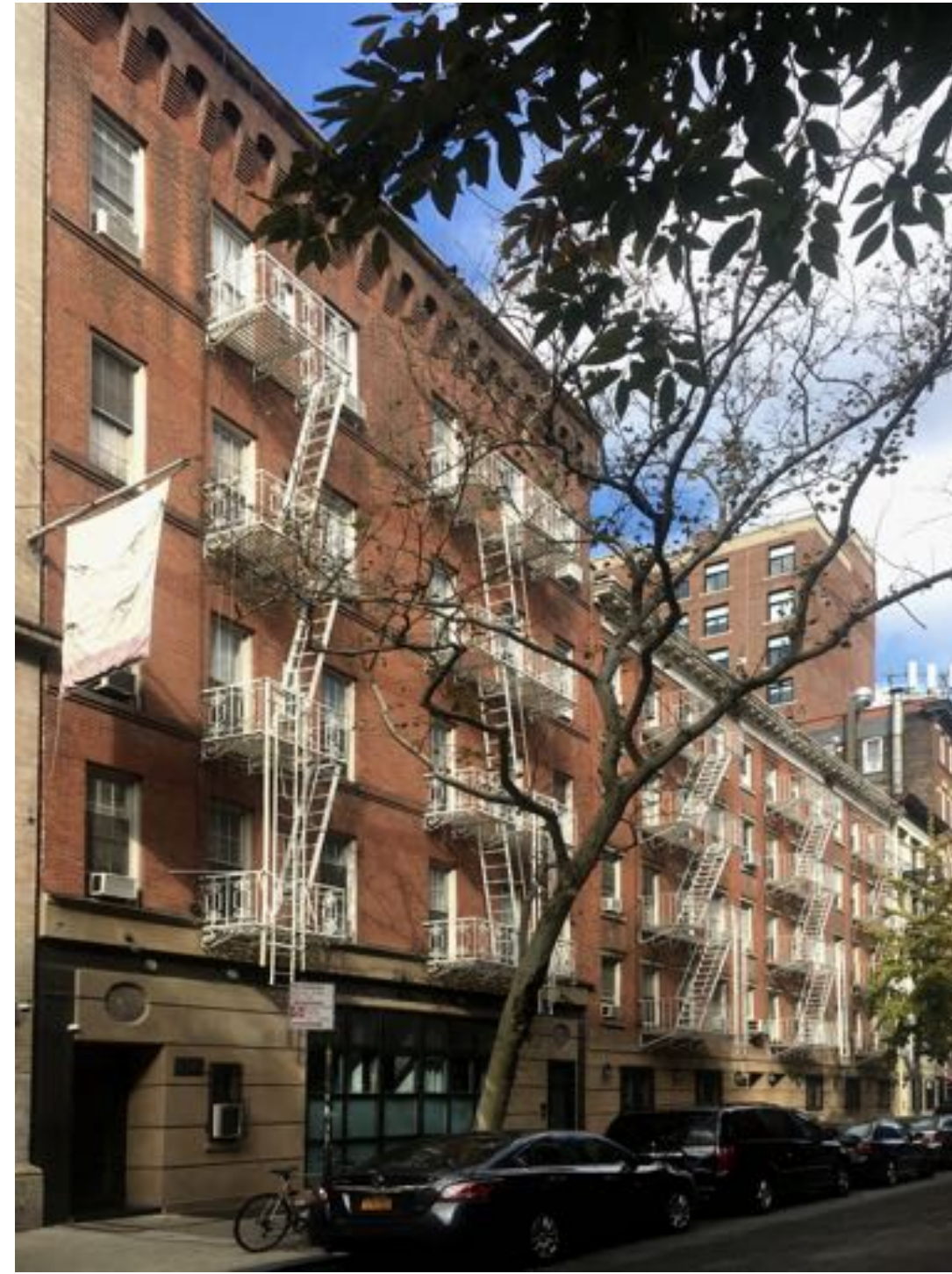
1 EXISTING STREET VIEW FROM SOUTH
