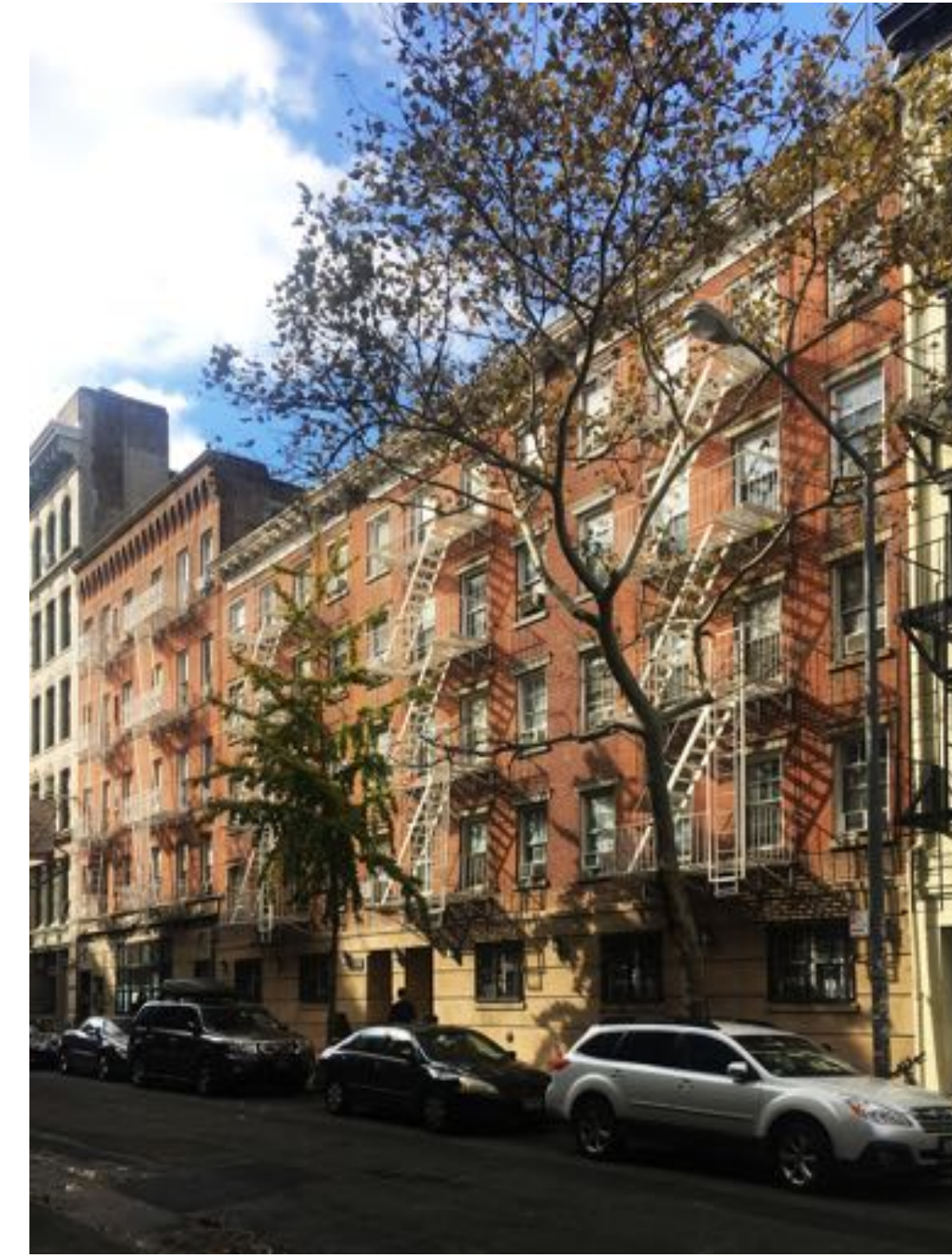
2 EXISTING STREET VIEW FROM NORTH
